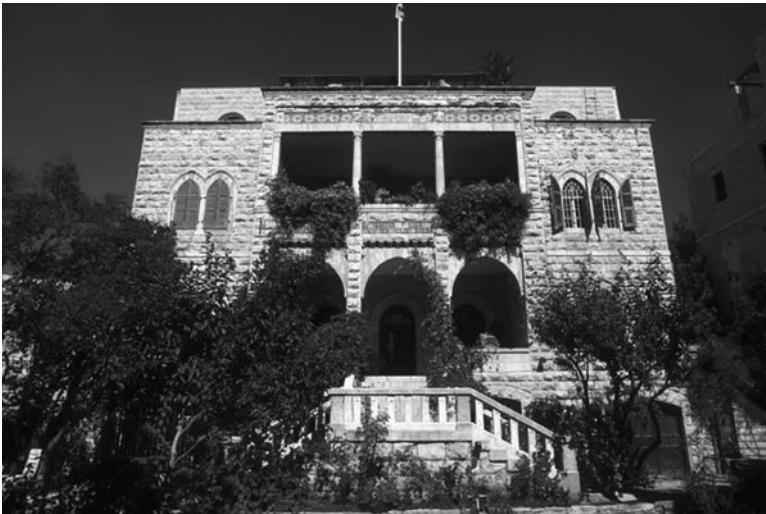
2. The Palestinian Bisharat family home in Talbieh, 2003. The structure was built in 1925 and appropriated by the new Israeli state in May 1948. Former Israeli Prime Minister Golda Meir occupied the home in the 1960s. Note the added-on third floor meant to look like part of an original whole.
