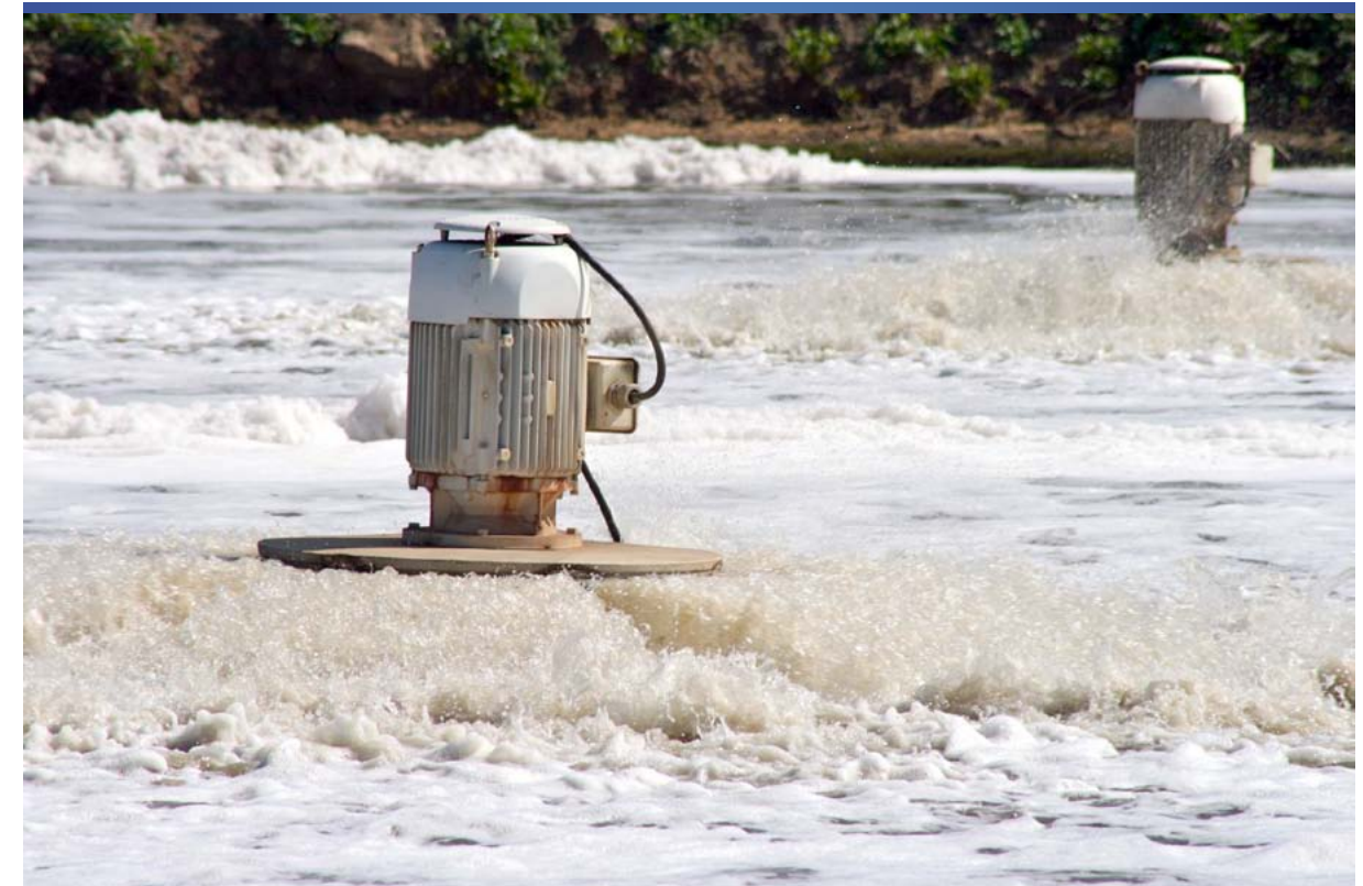
The wastewater treatment plant in Beit Lahiya, North Gaza governorate, has been operating beyond its capacity for many years. Wastewater that has received basic treatment flows into lagoons from where it then seeps into the groundwater. In North Gaza, Israel has prohibited the construction of sewage outlets into the sea, because of the risk of pollution that the partially treated wastewater poses to the southern beaches of Israel. The partially treated wastewater is thus forced back into the groundwater system, further polluting the Coastal Aquifer – Al-Haq©.
