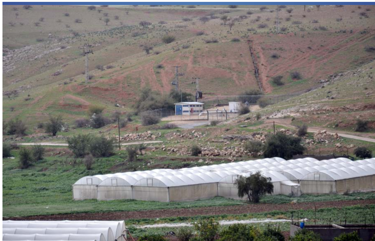
'Mekorot' pumping station, Jordan Valley – Tony Kane©.
