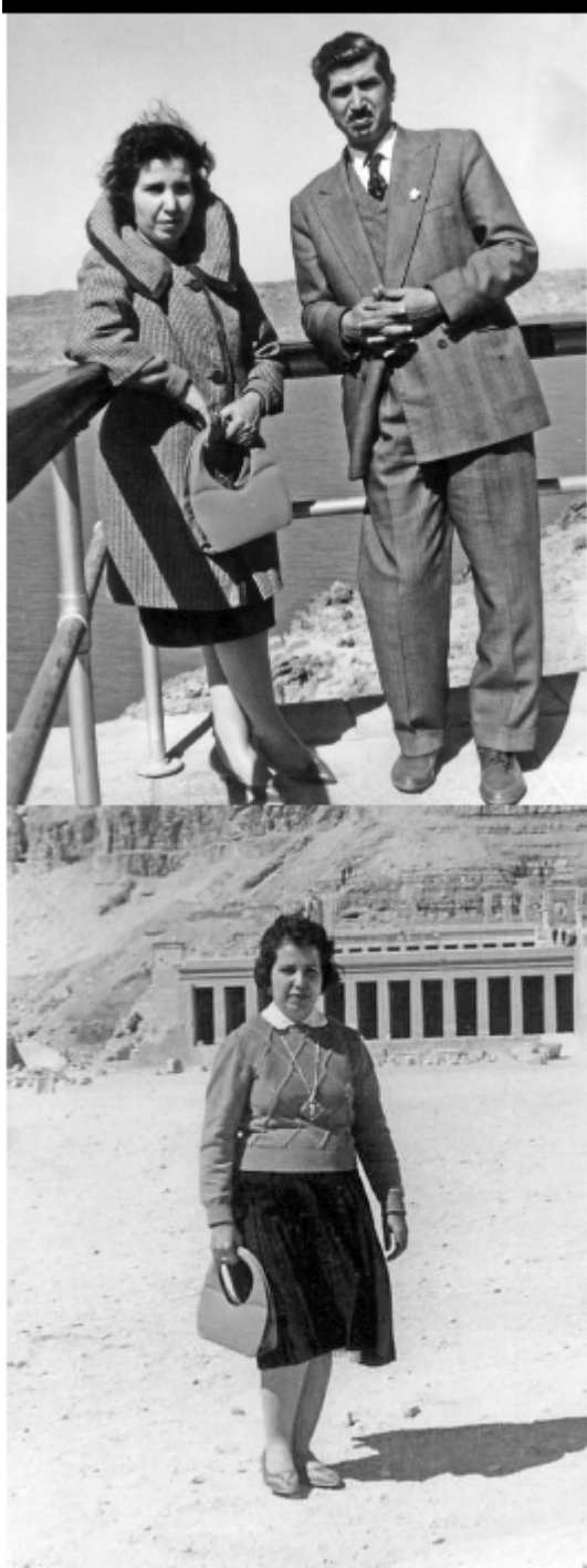
< Top: Madeeha Hafez Albatta with her husband Ibrahim Abu Sitta on their trip to Egypt for the conference in February 1961. The photo was taken at the construction site of the High Dam in Aswan. Photo courtesy of Madeeha's family.
