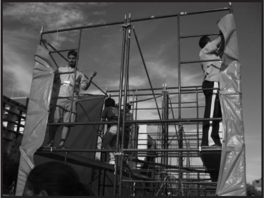
Mock wall construction, University of Arizona. (Courtesy UA SJP)
