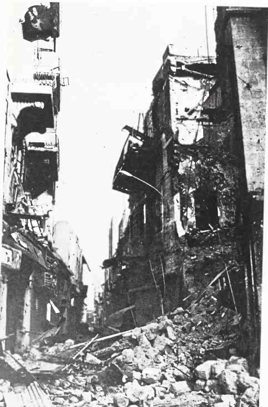
A street in Ashrafiyah after being bombed by the Syrians, 1978
