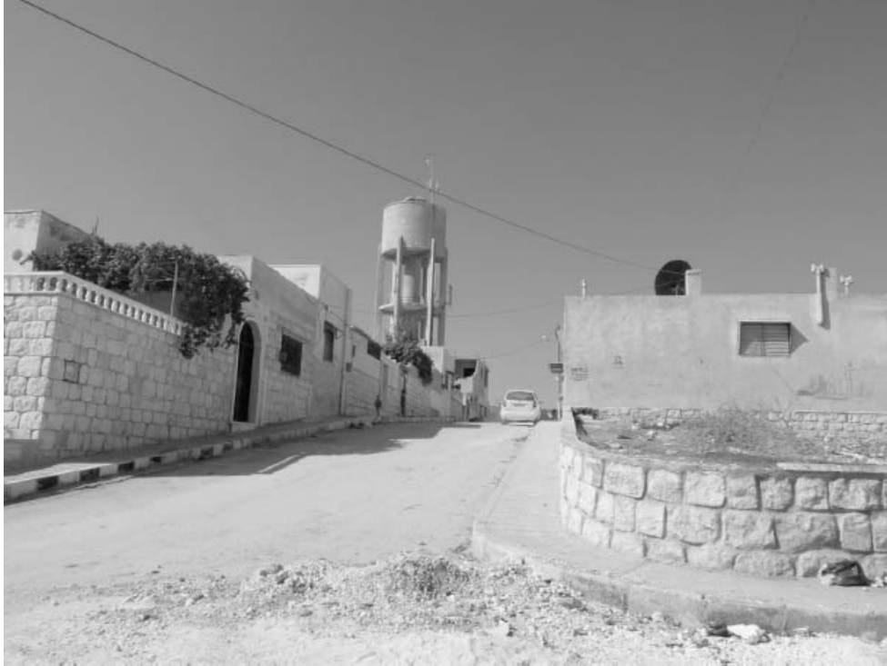
Figure 6.4. New water tower in Ein el Tal, 2011. Photograph courtesy of Lex Takkenberg.
