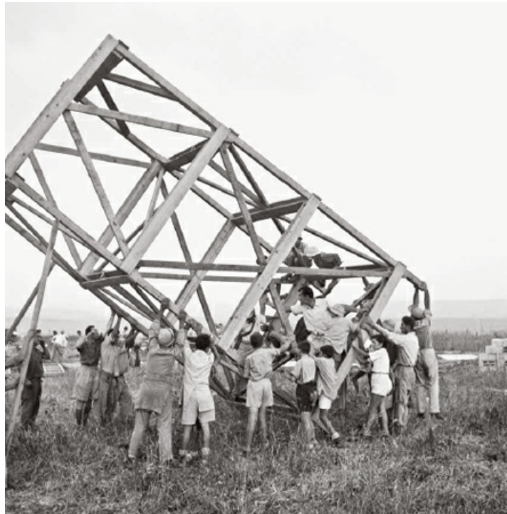
Men constructing a "tower and stockade" ( homa u-migdal ) settlement. Central Zionist Archives
