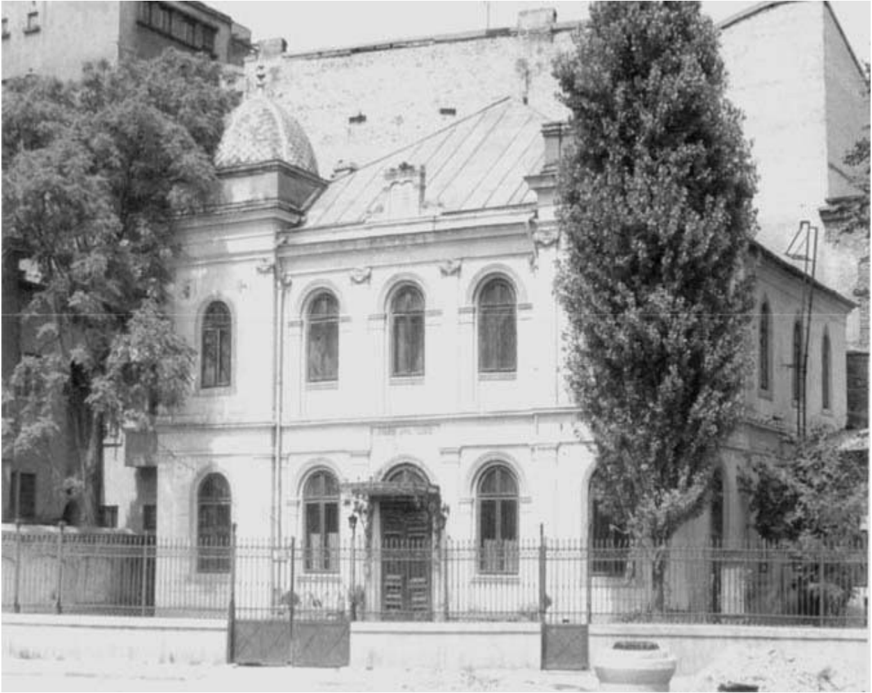
4. The Sephardic Synagogue in Bucharest before being demolished in August 1986.
