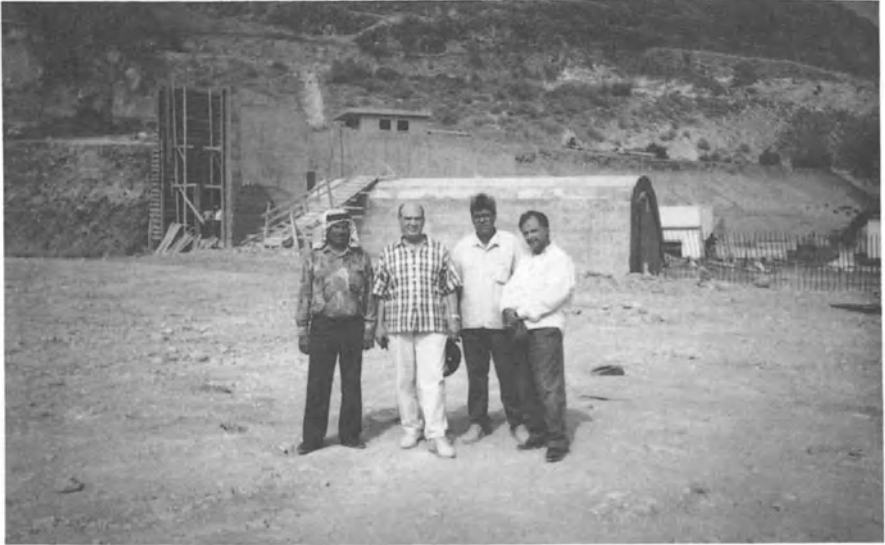
Figure (XII.2)- Picture of the Diversion Weir in Place
