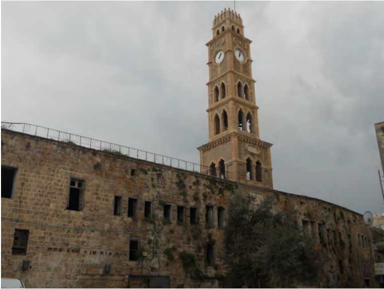
Outside of the khan (caravanserai) in the Old City of 'Akka
