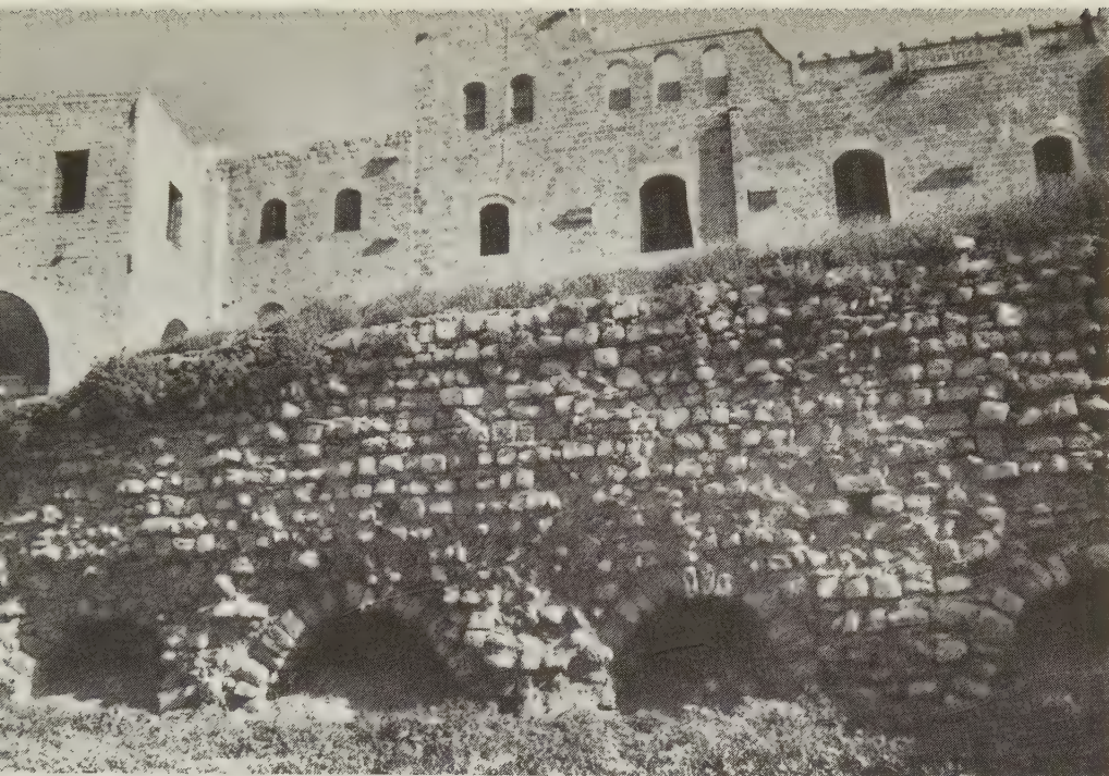
Remains of southern wall of Old Jaffa (Kark, 1977)
