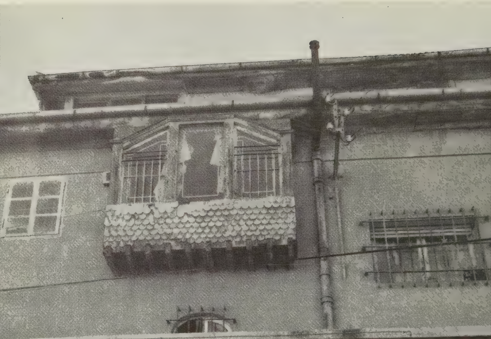
Early twentieth-century building, balcony embellished with wood (Kark, 1977)
