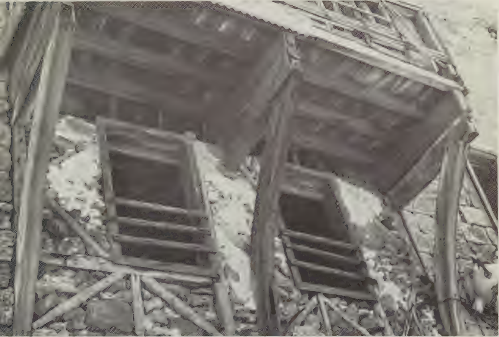
Construction of kurkar, filler and wood in Greek Orthodox Compound (Kark, 1977)
