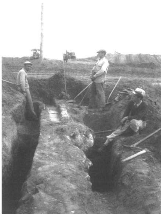
Figure 16. Rishpon, 1951. Hired excavation workers, before the relief work system. (IAA 1302)
