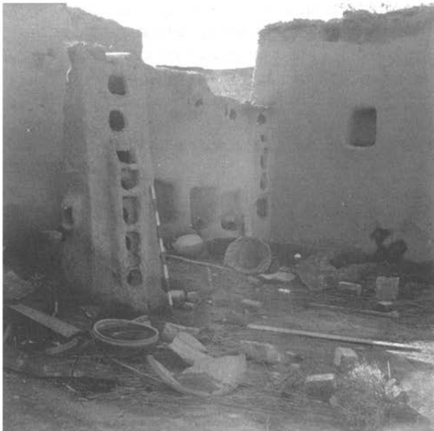
Figure 6. Abandoned village of Khartiyeh, November 1948. Mud houses with tools. (Photograph by Ory, IAA 143)
