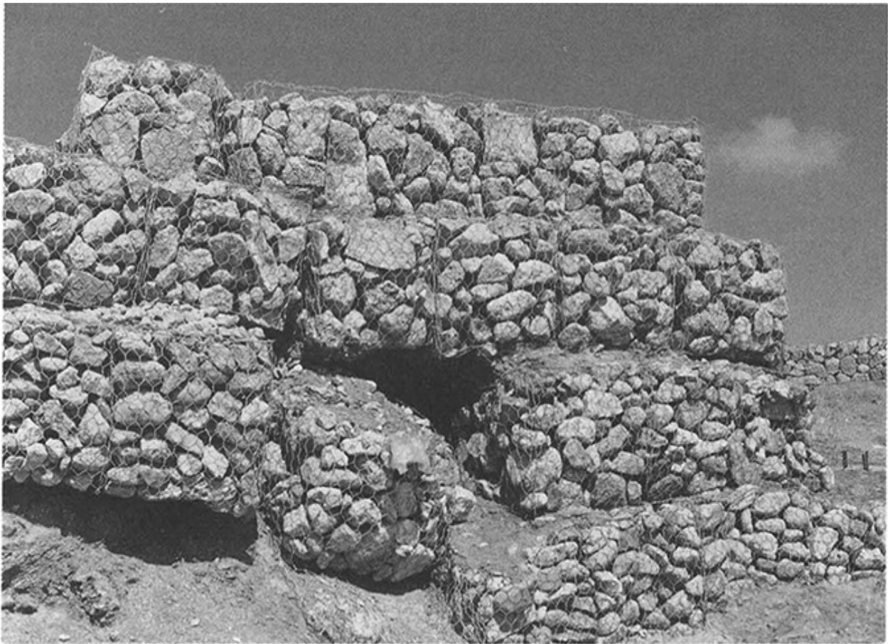
An Israeli bunker fortified with rocks in wire-mesh baskets (author's photo)
