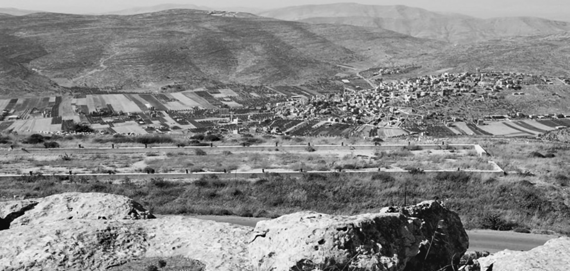
FIGURE 3.9. The foundations for the chicken coop at the Three Seas Lookout. The coop is situated on a high hill overlooking Beit Furik, a Palestinian village at the outskirts of Nablus, seen here in the background. Photo by author.
