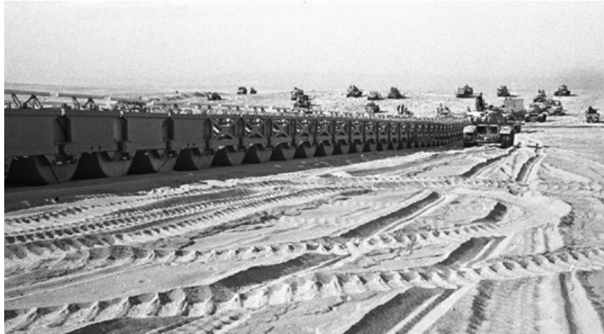
Grappling with the monster. Tanks drag the 180-meter-long rolling bridge toward the canal. (illustration credit ill.29 )
