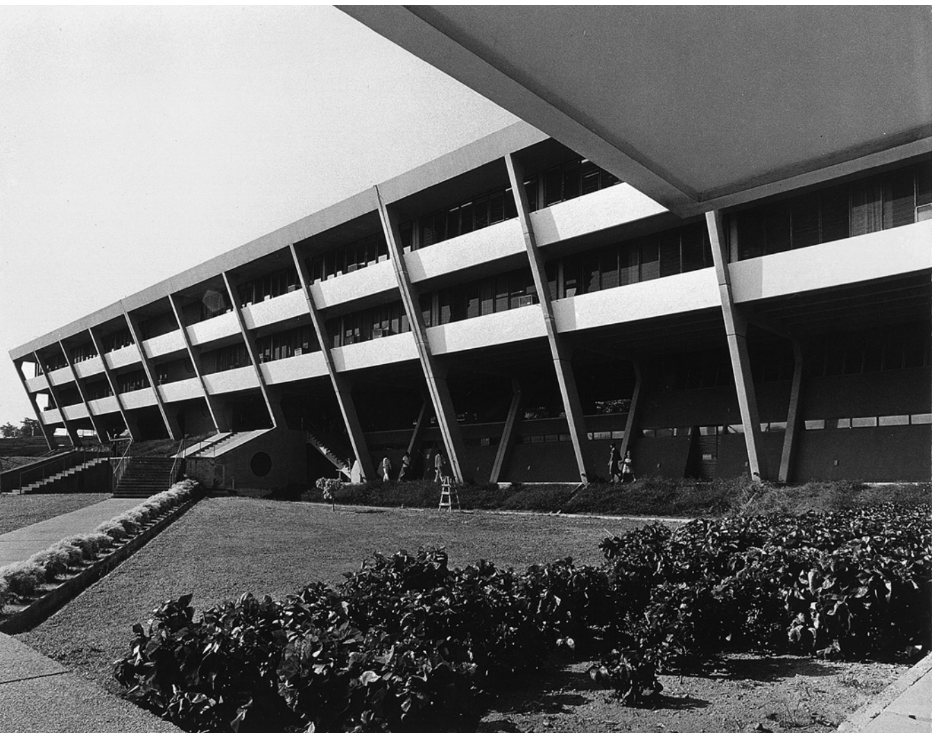
FIGURE 4.12 Harold Rubin, Faculty of Education, southern facade, University of Ife, early 1970s. Courtesy of Amos Spitz.
