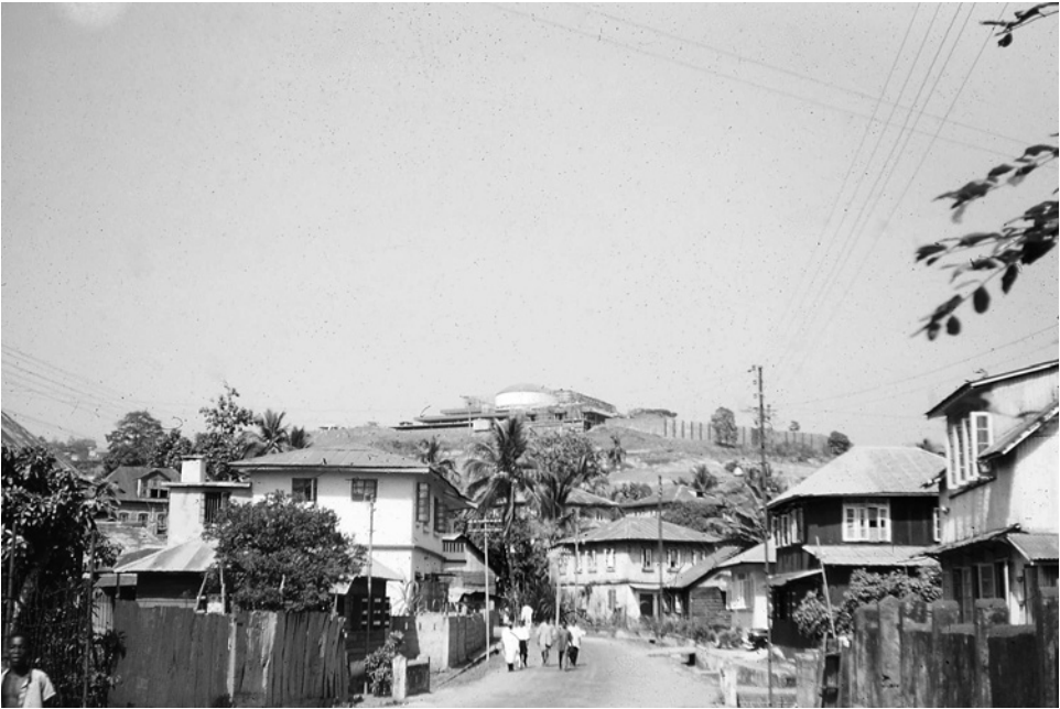
FIGURE 1.7 The Sierra Leone parliament under construction, Tower Hill, Freetown, April 1961. Courtesy of the Azrieli Architectural Archive; Ram Karmi collection, 8267357058013.
