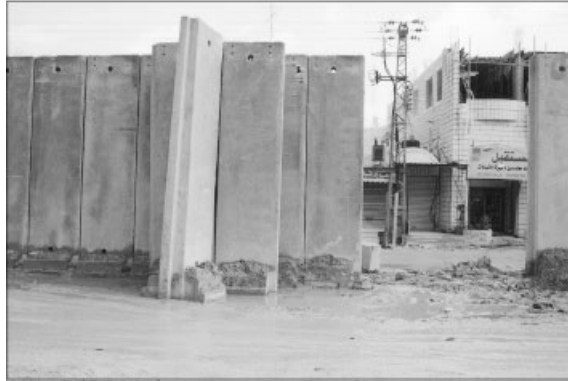
Wall under construction near Jerusalem. Photo by author.
