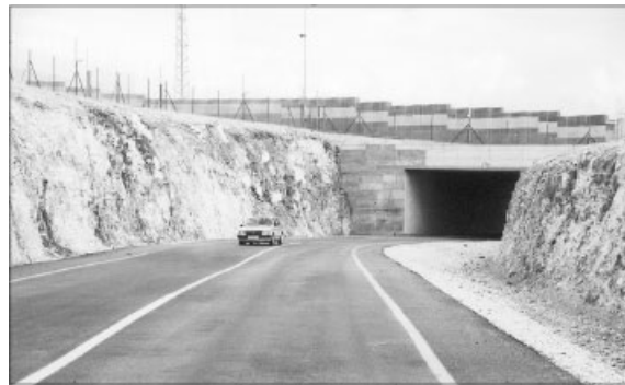
Tunnel for Palestinians beneath Israeli bypass road, West Bank. Photo by author.
