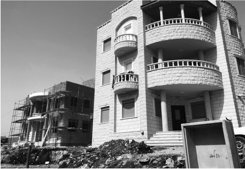
5 A home under construction next to one occupied
