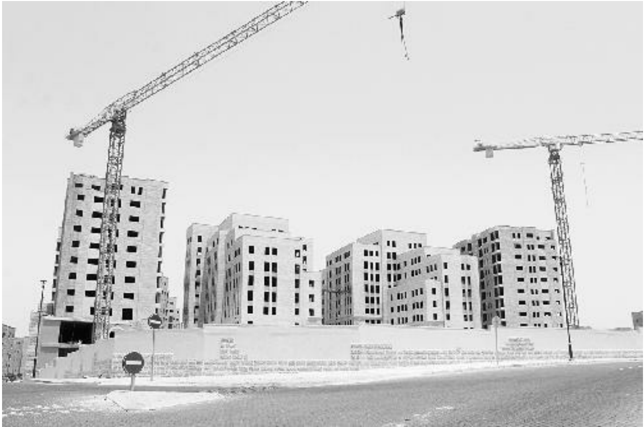
FIGURE 1.13 Construction in 2017. Photo by Léopold Lambert for The Funambulist .
