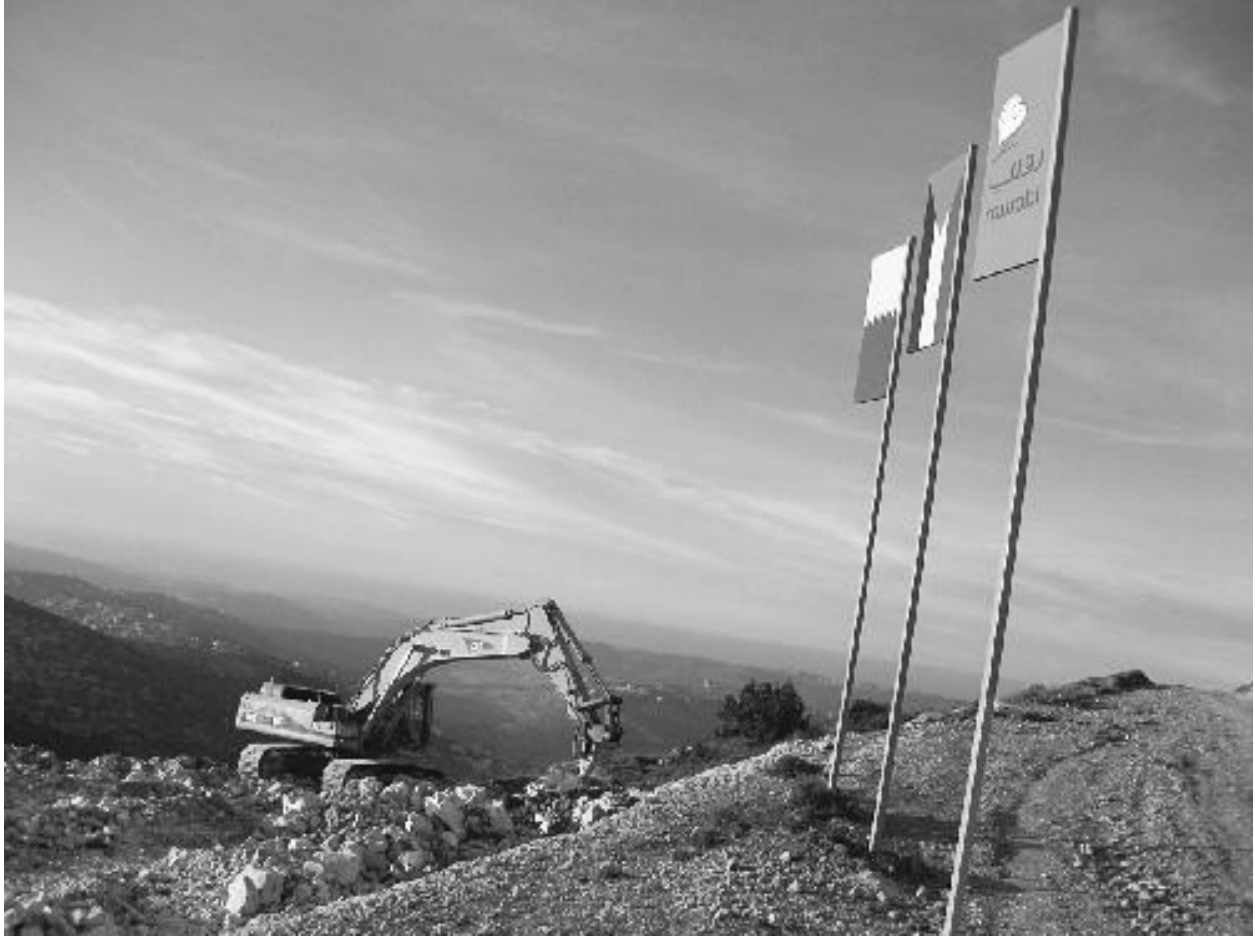
FIGURE 1.5 Rawabi in January 2010. Photo by the author.
