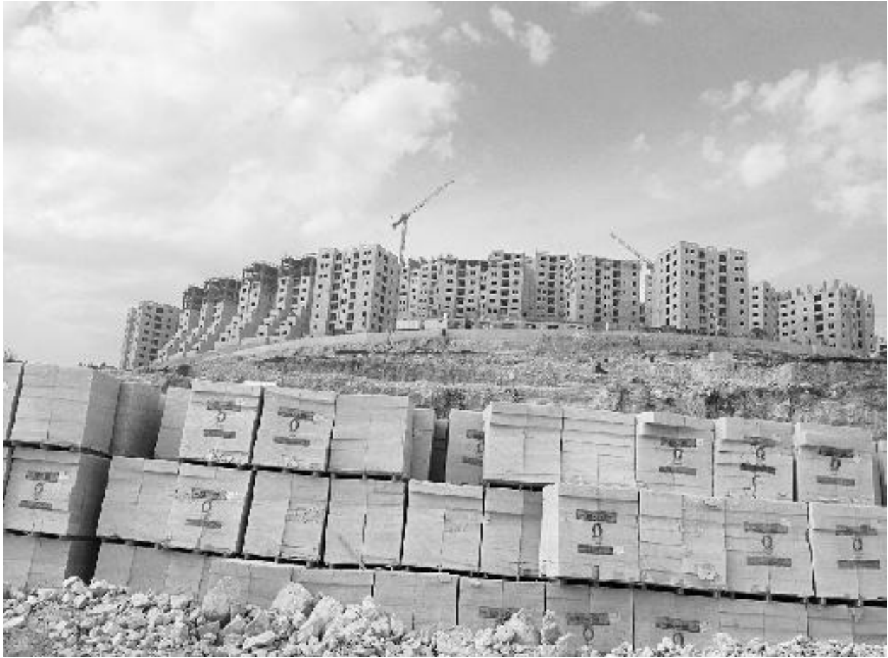
FIGURE 1.9 Construction in 2013. Photo by the author.
